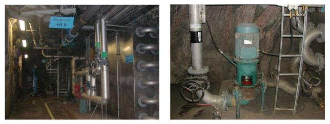
Figure 7. On the left – the heat exchanger coil below anaerobic digester 5 at Henriksdal. On the right – the dosing point (at the bottom on the right) for the LiCl solution.
