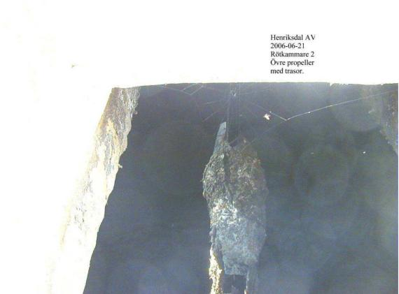
Figure 25. The upper propeller blade is clogged with shreds.
