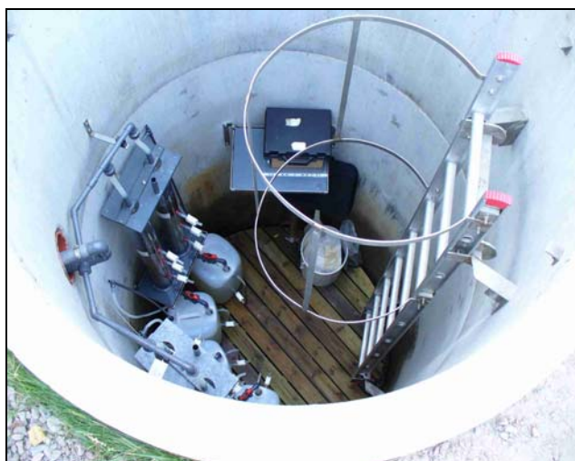
Figure 3. Column set-up in reactive filter manhole
